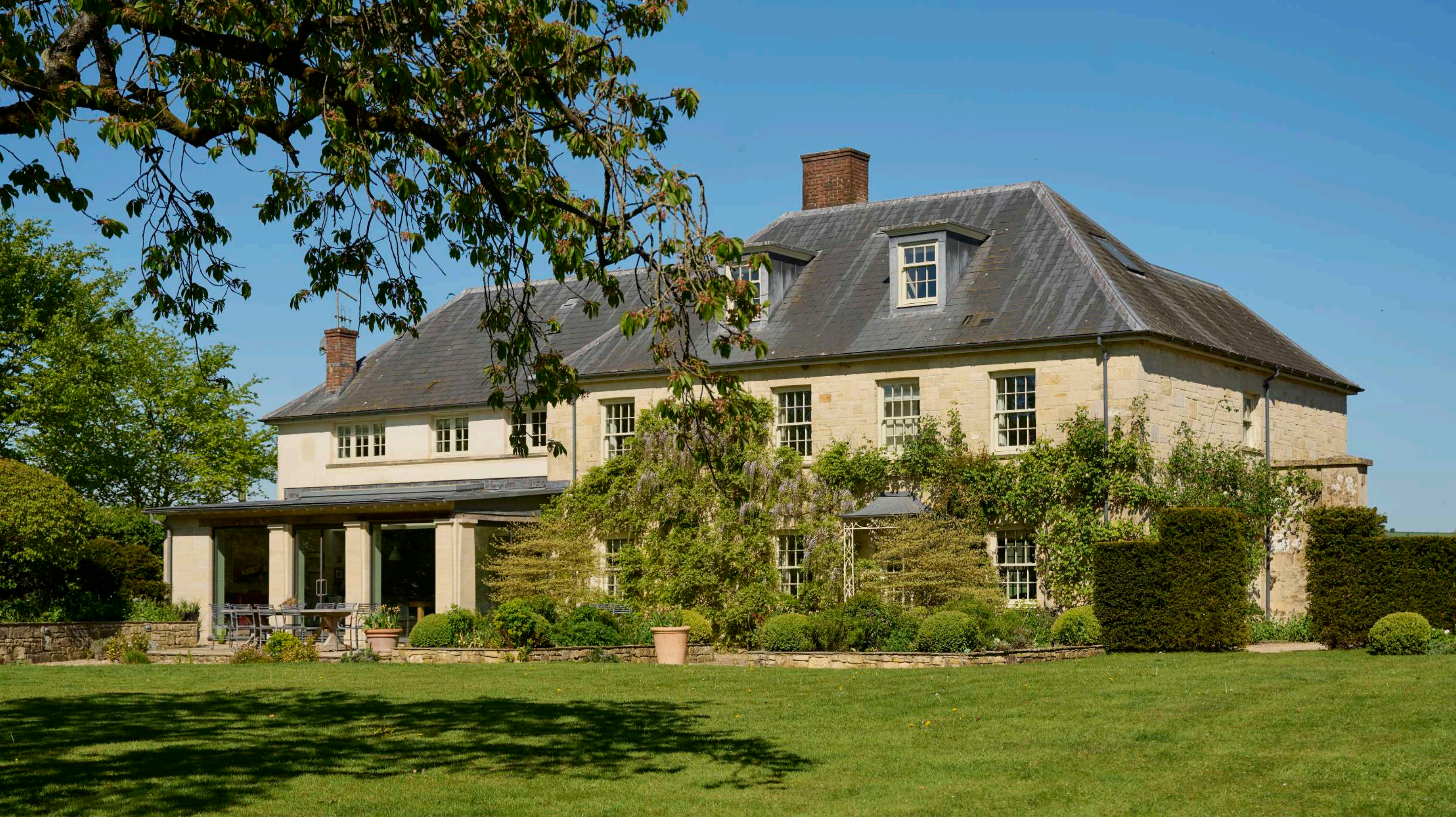
DRUM HOUSE Tisbury, Wiltshire
